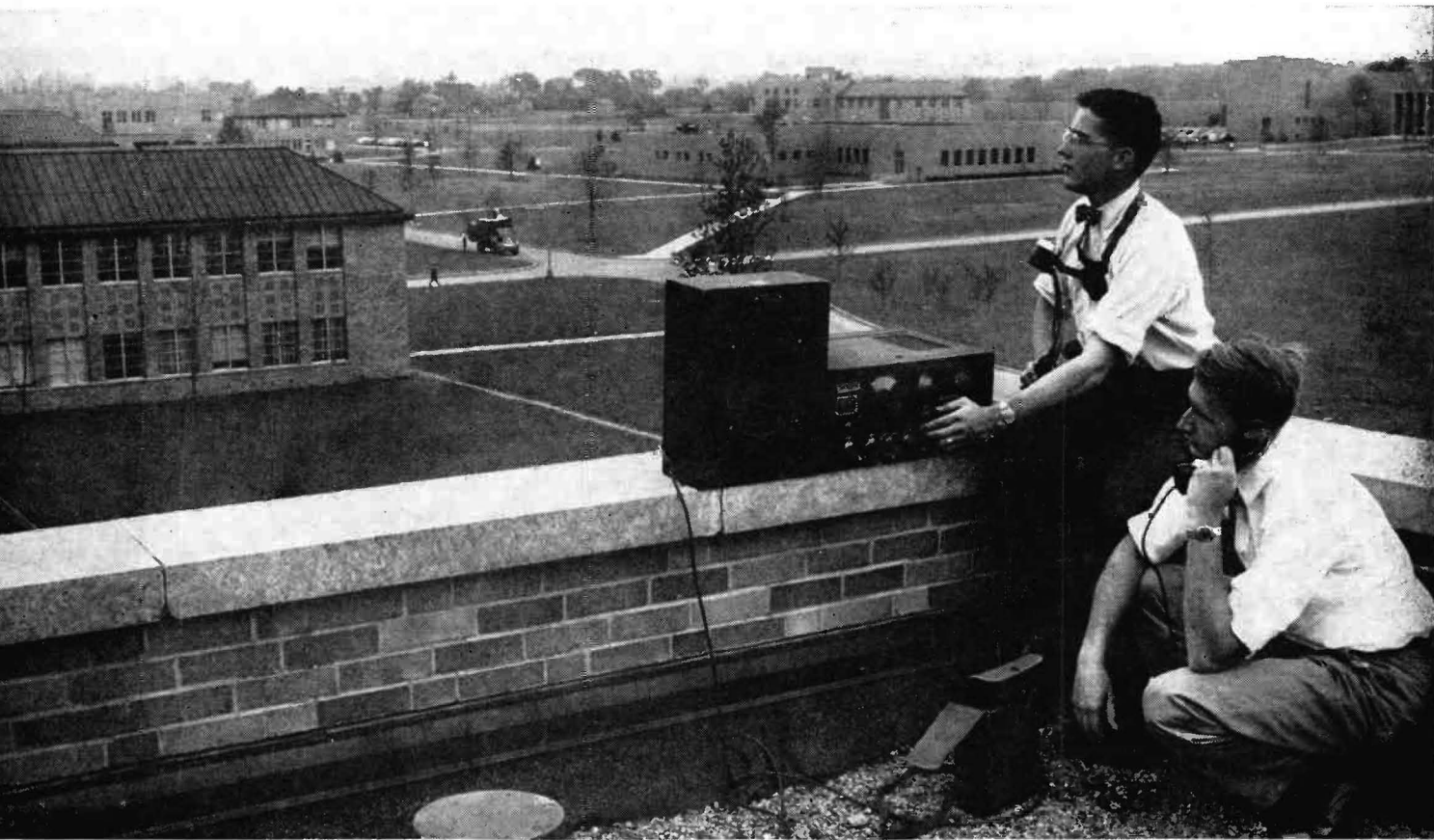
ROOFTOP PANORAMA —Radio communication test point on Transmitter Building roof, with land-line telephone "just in case"
