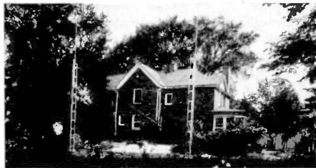
Fig. 2—View of the building and antenna towers of the monitoring station at Deerfield, Illinois, looking from the transmitters.
