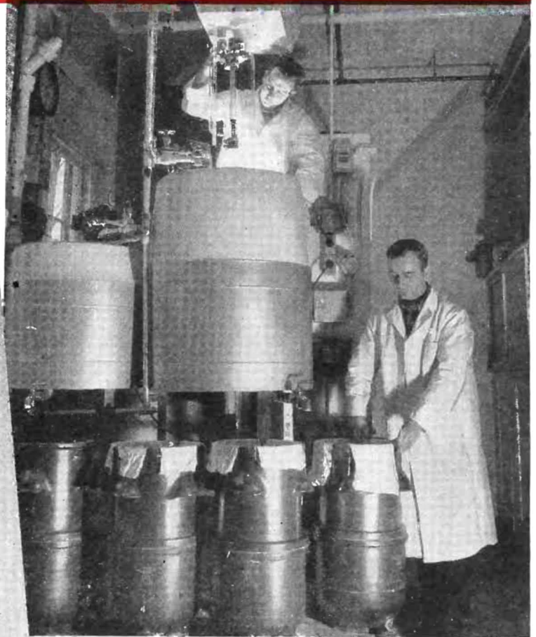
First floor of Hytron chemical precipitation system. Note the flow meter, precipitation tanks, and ceramic vacuum filters. Spotless cleanliness is vital to avoid contamination of carbonates precipitated for cathode coatings.
