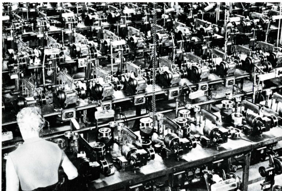
Through various drawing methods and annealing steps, Sylvania can produce different physical characteristics in wire of a given size. Above, general view of tungsten wire drawing department.
