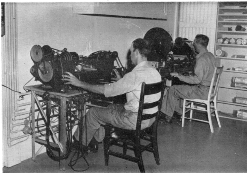
Glass Lathe Sealing
