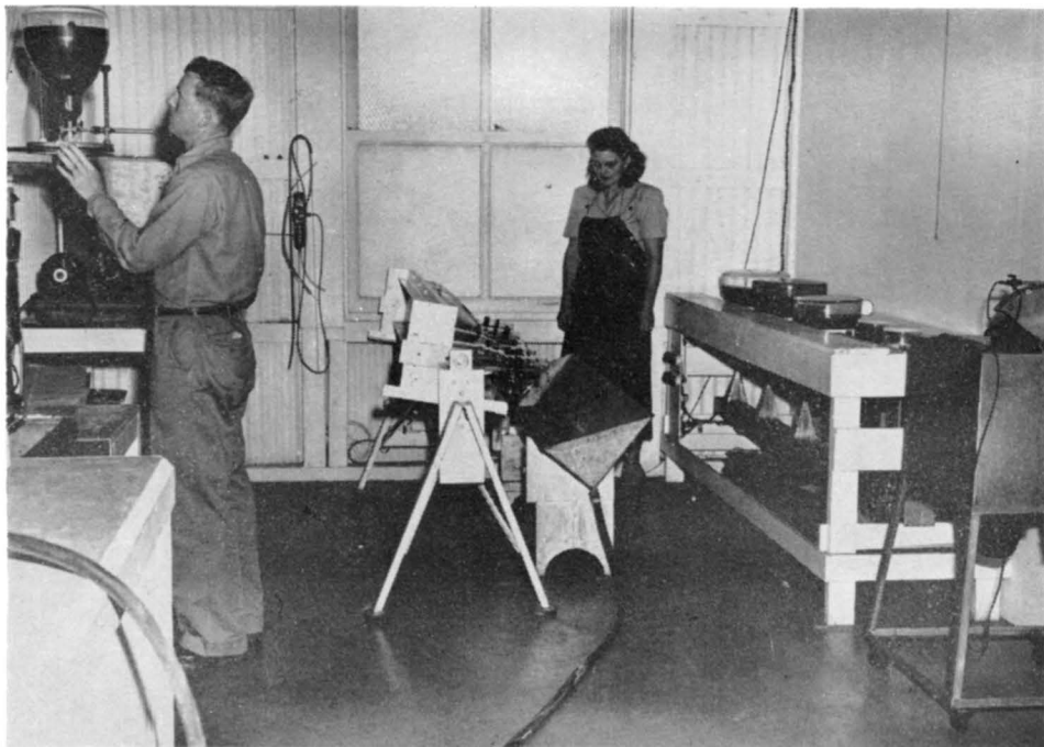
Phosphor Settling — Inner Wall CRT Coating
